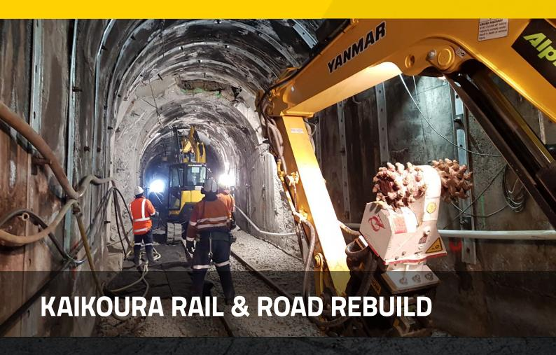
The Kaikoura earthquake caused substantial damage to the Christchurch to Picton rail line and tunnels, which are over 100 years old. The tunnels suffered substantial damage from rock falls, cracking and general weakening. Some sections had vertical and transverse movement in excess of 500mm, from transverse faults running through the tunnels.
