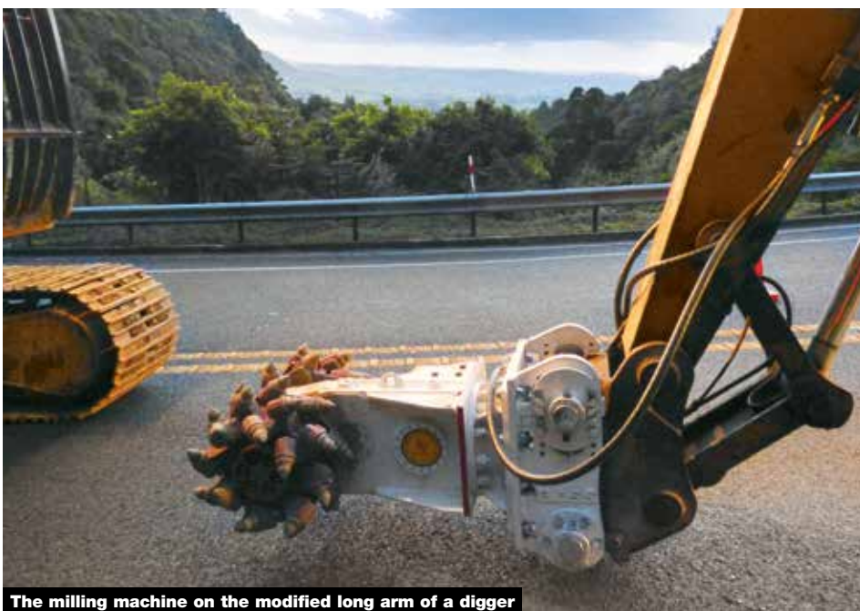
The milling machine on the modified long arm of a digger
